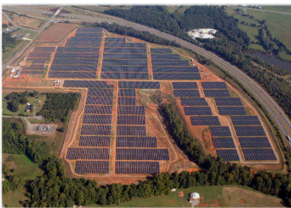
Maiden solar photovoltaic array
